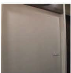
Step-1: Provide a dry & levelled wall surface
