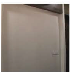
Step-1: Provide a dry & levelled wall surface
