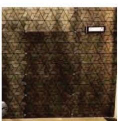
Step-6: Use spacers for interlocking panels
